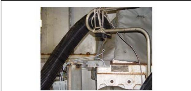
Photo 2: Growth probes at inlet end.
