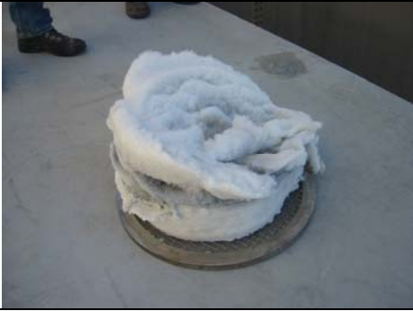
Photo 6: Silencer packing material retrieved from downstream screens prior to aeration tank
